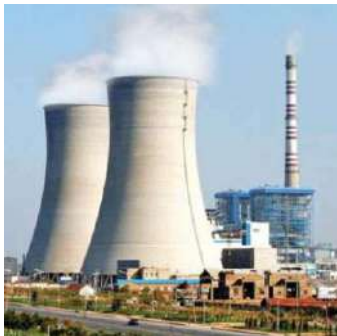
ENERGY / THERMAL POWER
